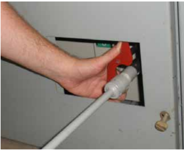
Figure 19 - Racking Through Sliding Panel
